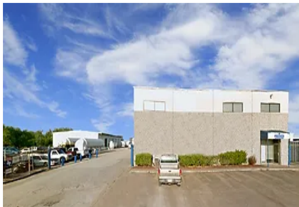
EXTERIOR MAIN BLDG
