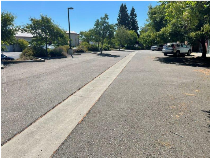
13. Eastern parking area: concrete drainage swale manages storm water.
