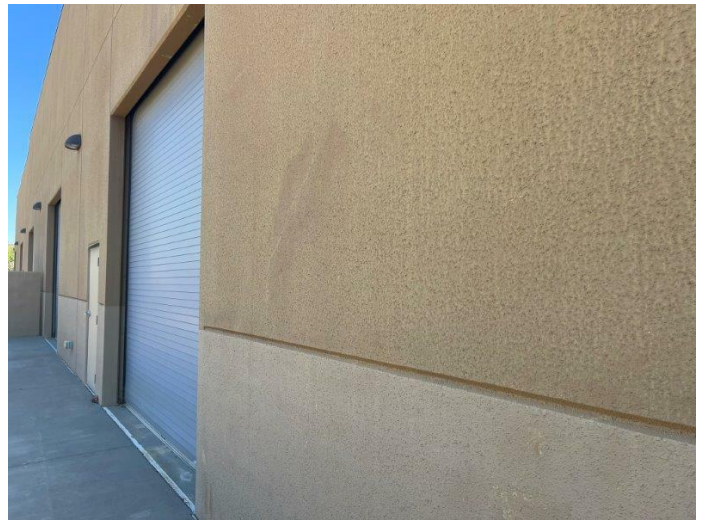
20. Primary facade material is painted concrete tilt-up panel.
