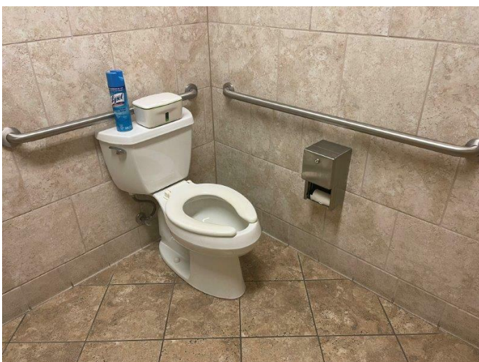
47. Warehouse restroom: fixtures and finishes.
