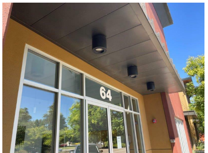
18. Lighting at soffits above entries.
