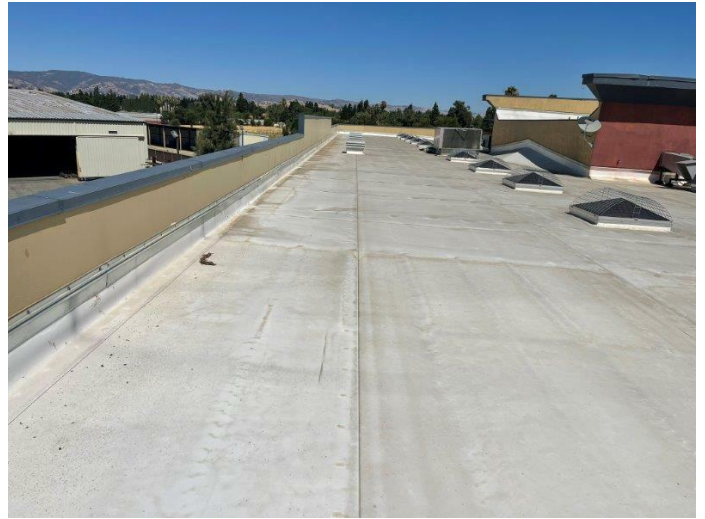
26. Western rooftop field, looking northerly.
