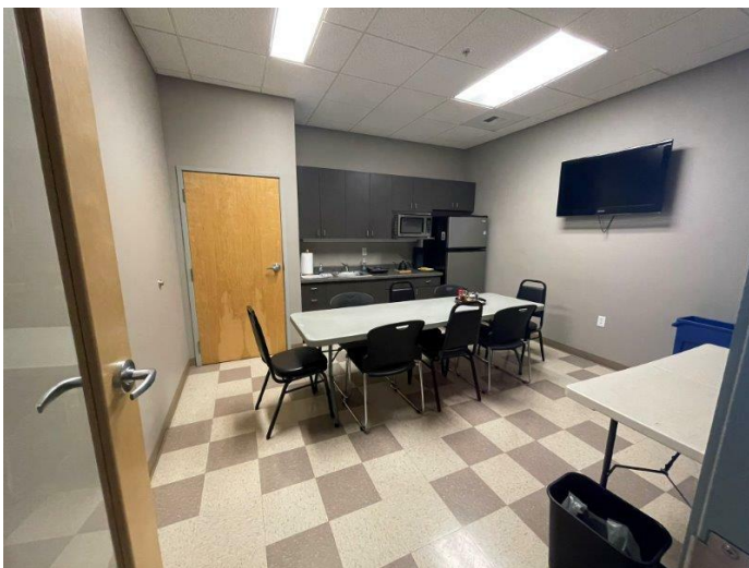
41. Second floor, break room: floor, wall, and ceiling finishes.
