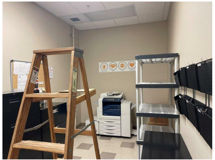
40. Second floor, support room: floor, wall, and ceiling finishes.
