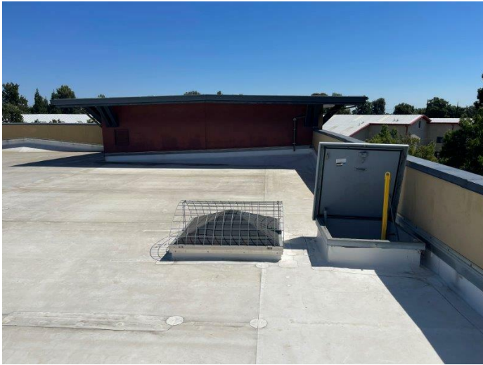
25. Southern rooftop field, looking easterly.
