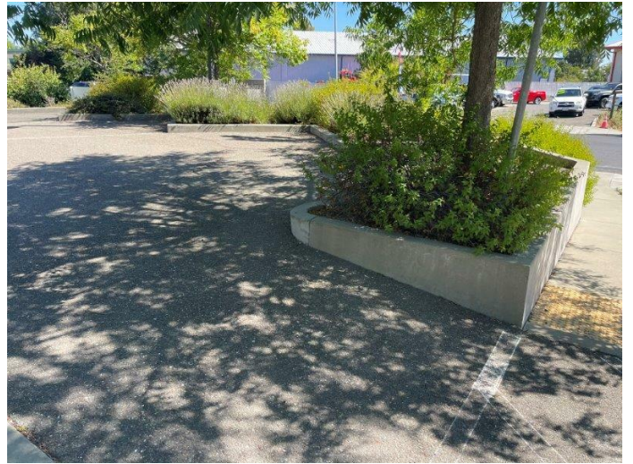
14. Asphalt paving and retaining walls for landscaping.
