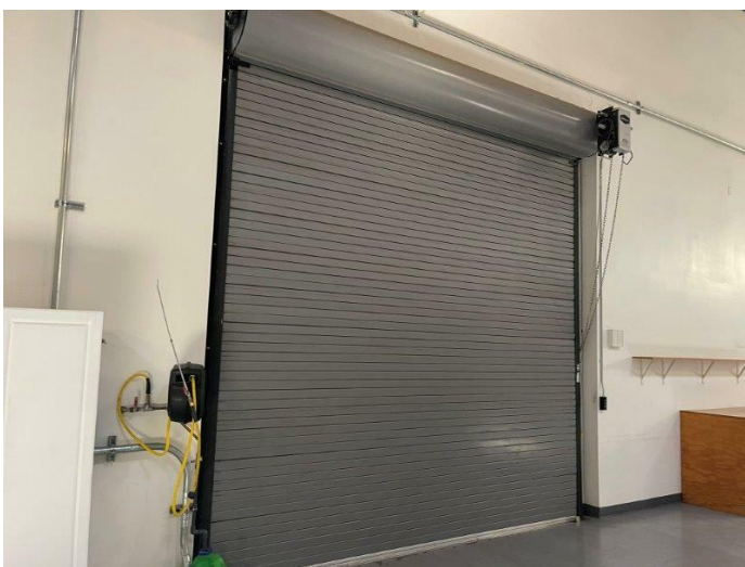
23. The property is provided with six self-coiling metal doors.
