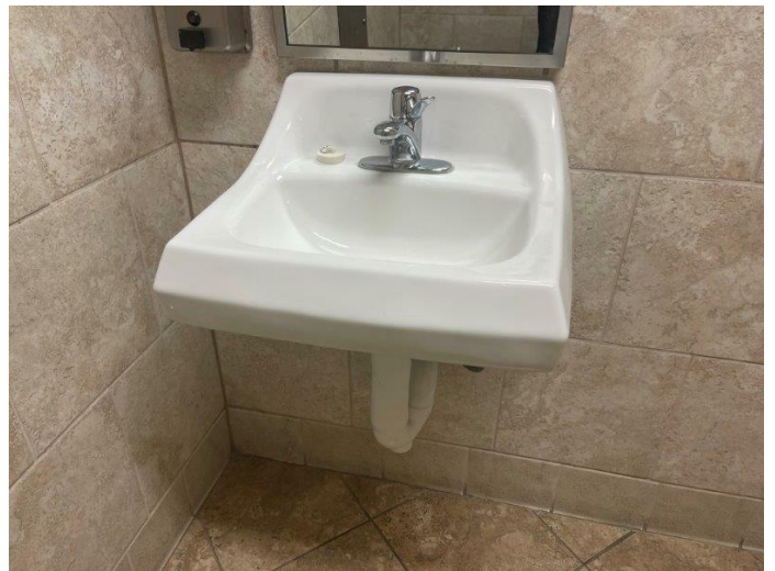
46. Warehouse restroom: fixtures and finishes.
