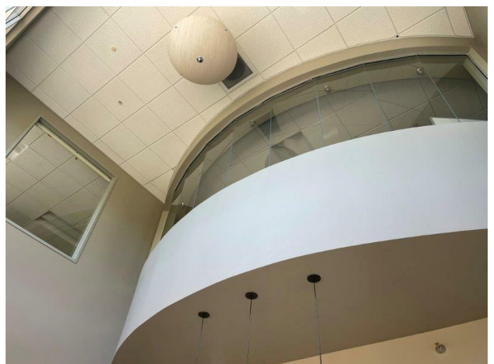
36. Entrance lobby ceiling and mezzanine area: finishes.
