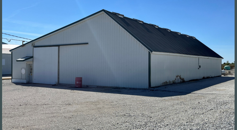
4,632 SF Storage Building
