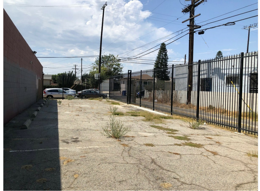
Interior fenced parking lot #2 w/access to bldg
