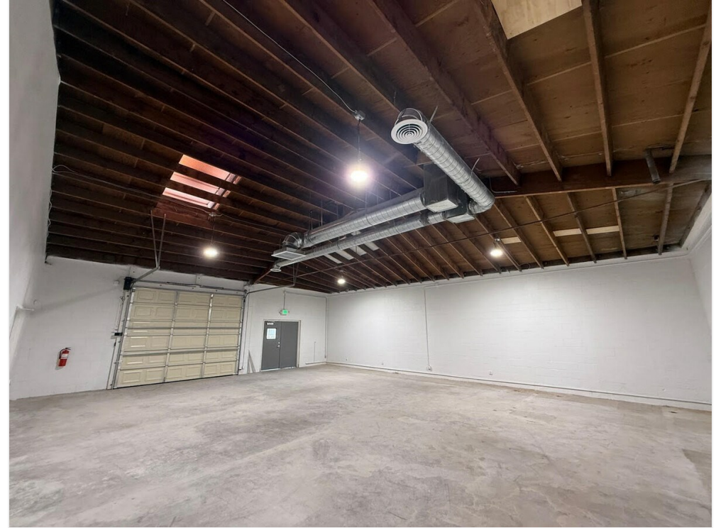
Interior view with ground level door
