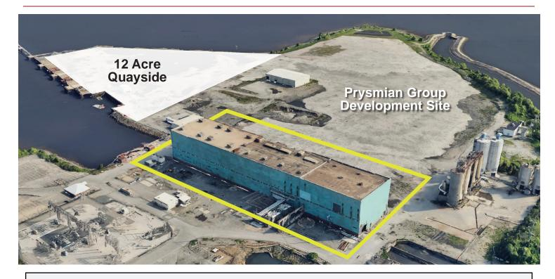
Formerly used as a crane bay for a coal power plant, this building has 100-ft ceilings, two 100-ton cranes, and up to 15 acres of land available for development.
