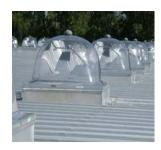
**Solar Tracking Skylights:** Solar Tracking Skylights consist of highly reflective mirror panels within a clear plastic enclosure, which move continuously to follow the sun's position in the sky. By aligning to the exact position of the sun, the mirrors reflect light down into the space that would be otherwise lost due to the low incident angle of the sun through much of the day.
