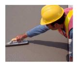
**Helix Concrete:** Polytorx Helix steel fiber concrete requires 20% less pour. Polytorx Helix concrete is a Michigan developed and manufactured product. Helix is high performance, optimized steel for use in the reinforcement of concrete. Helix is short, twisted and polygonal shaped wires that are added to concrete during mixing resulting in less concrete needed.
