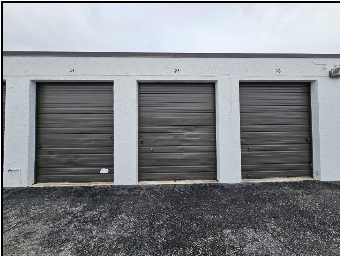
Typical 150 SF or 200 SF unit on the west side with one overhead door
