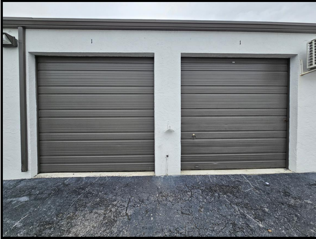
Typical 775 SF unit on east side with 2 side by side overhead doors
