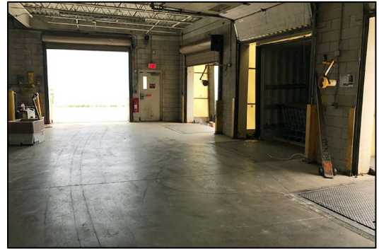
Drive-in door adjacent to docks
