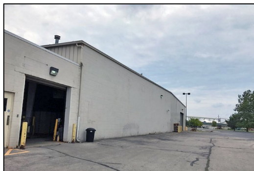
Eastern Elevation - Supply Warehouse
