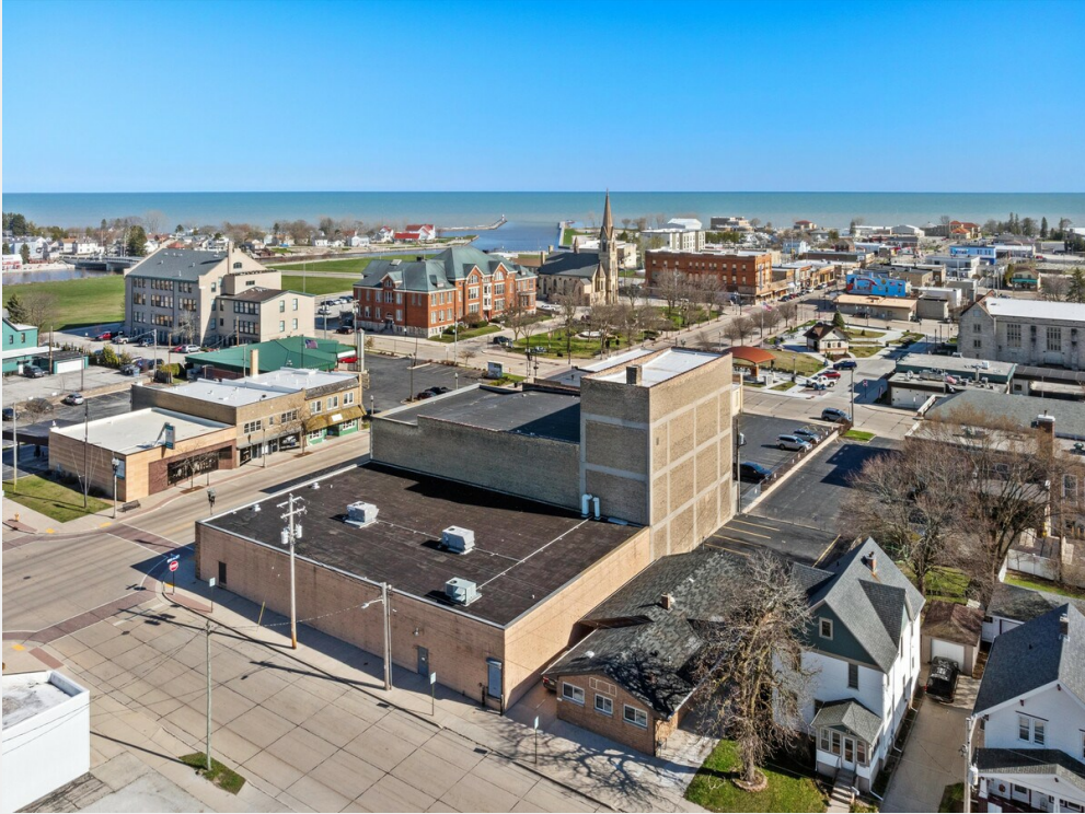
Aerial View of north and west side of the building
