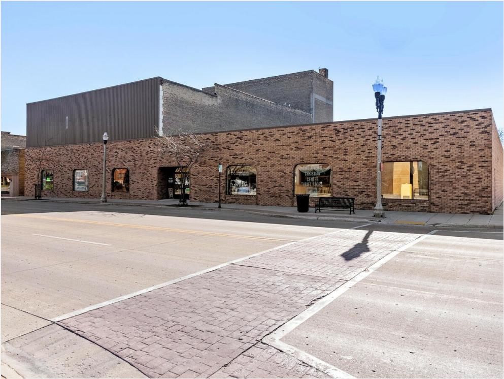
Main Front View of the building
