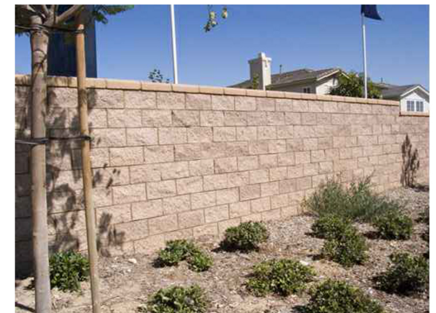
I MASONRY WALL
