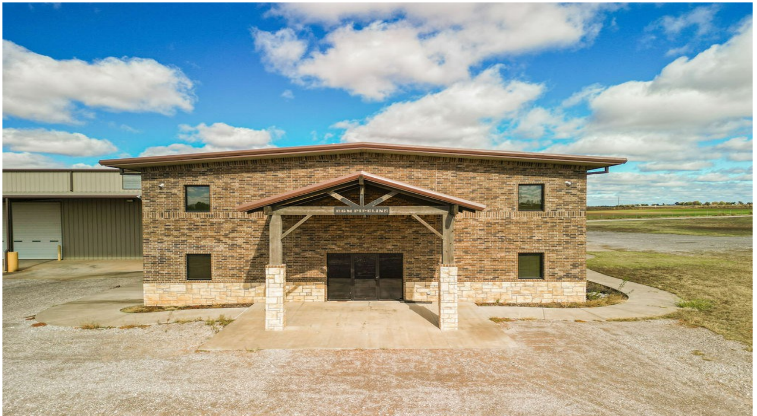
South Office Entry
