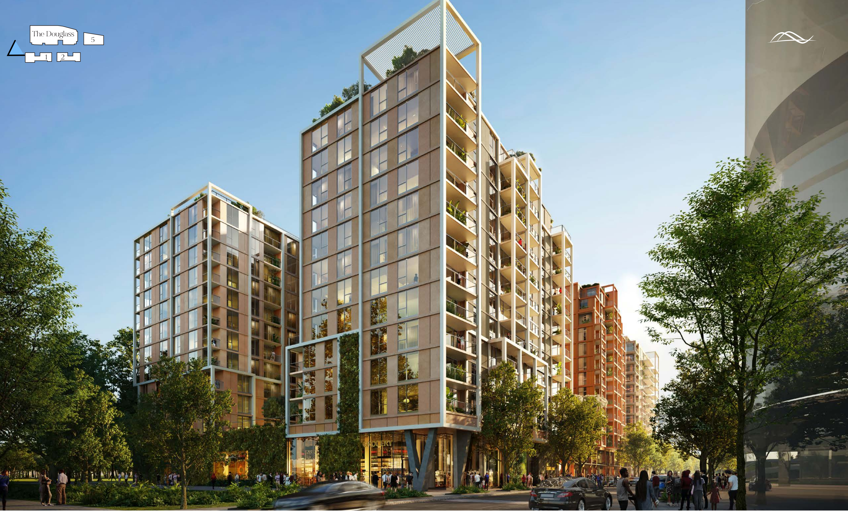
The Douglass: SW Corner of Howard Road
