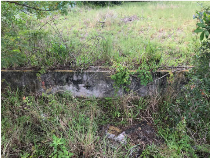
Looking at block wall that intersects subject property.
