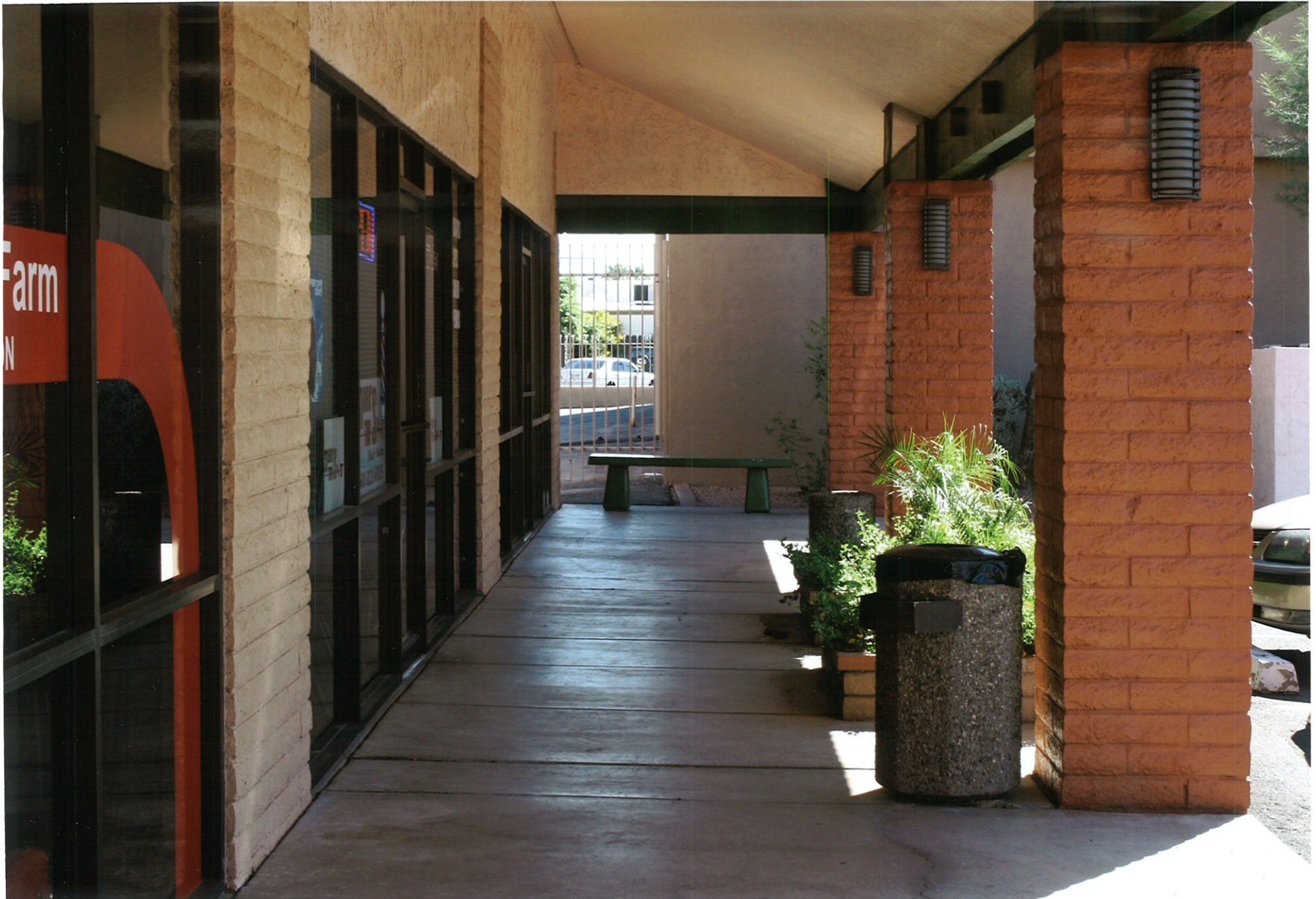
Walkway Looking East
