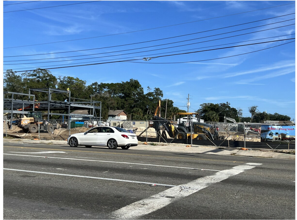
G - WaWa Construction Across Street
