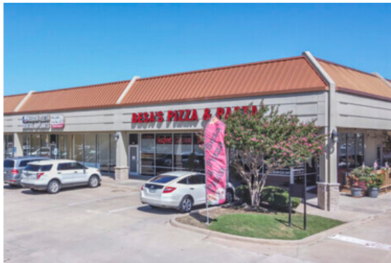
14856 PRESTON ROAD BUILDING 1
