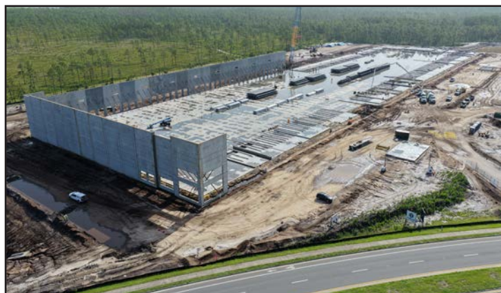
CONSTRUCTION PROGRESS - WALL TILTING
