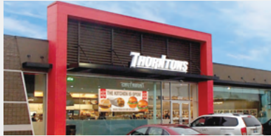
New Thorntons Gas Station
