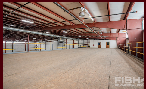
MEZZANINE WITH OFFICES
