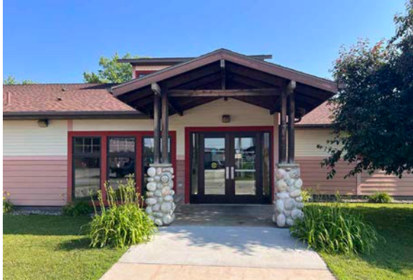
Front/South Side of Bldg - Main Entrance
