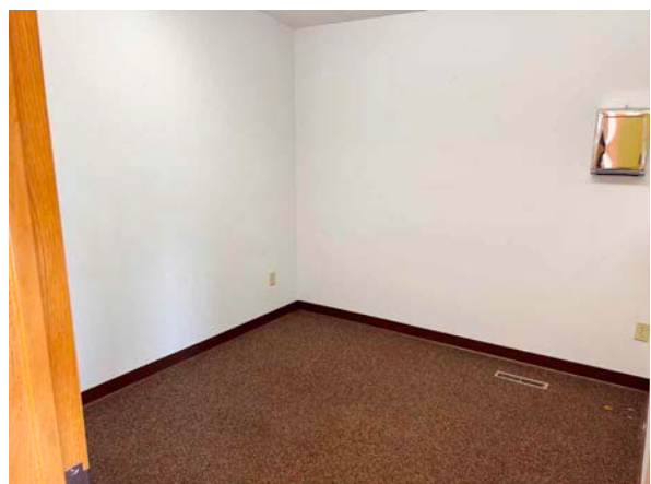
East Office - Office
