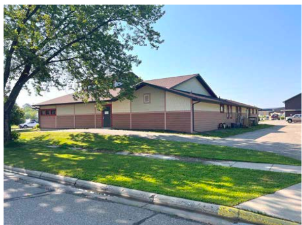
Complex - North & West Side of Building
