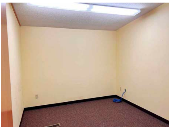
East Office - Office
