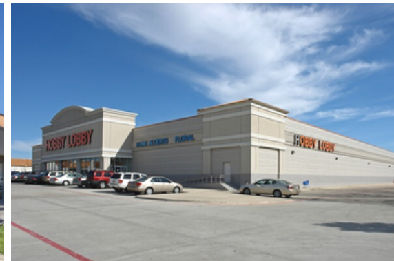
14858 PRESTON ROAD BUILDING 3 | HOBBY LOBBY
