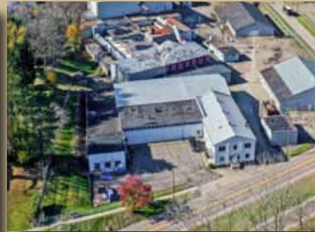
Aerial View (Looking West)
