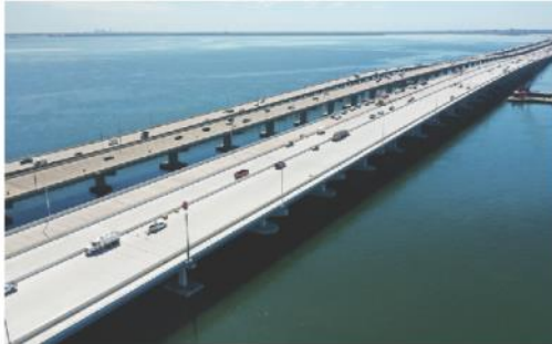
HOWARD FRANKLAND BRIDGE I-275
