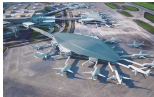
TAMPA INTERNATIONAL AIRPORT AIRSIDE D
