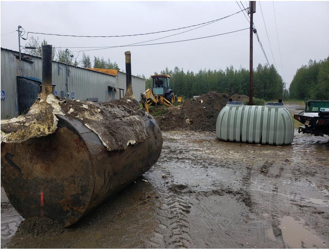
Photograph 17: Septic tank replacement project underway
