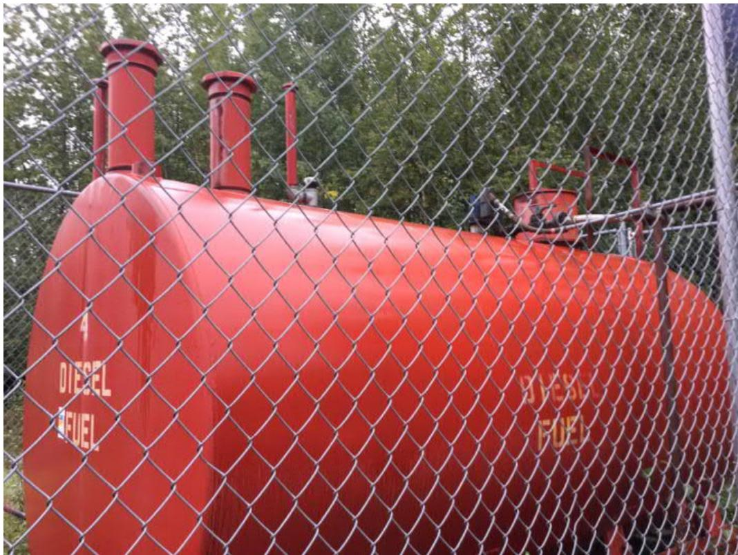
Photograph 13: 10,000-gallon diesel fuel AST
