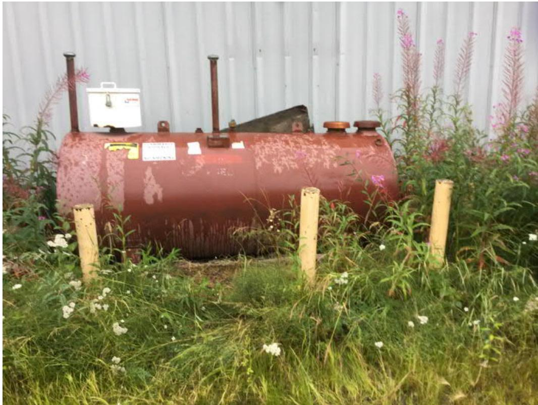
Photograph 15: Heating oil AST on building north side
