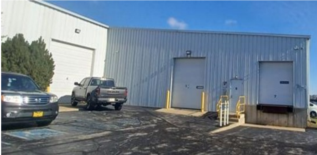
Overhead Doors, Dock
