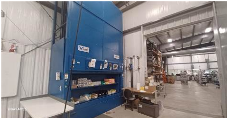
Manufacturing Area, view of interior door/fire door
