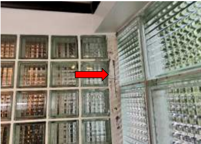
DETERIORATED/MISSING GROUT
