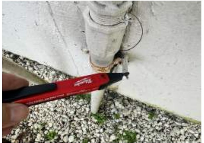
EXPOSED WIRES
