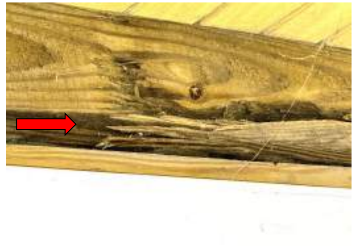
DAMAGED RAFTER
