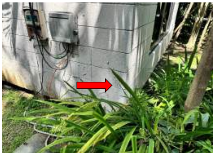
STRUCTURAL SETTLEMENT/CRACKING
