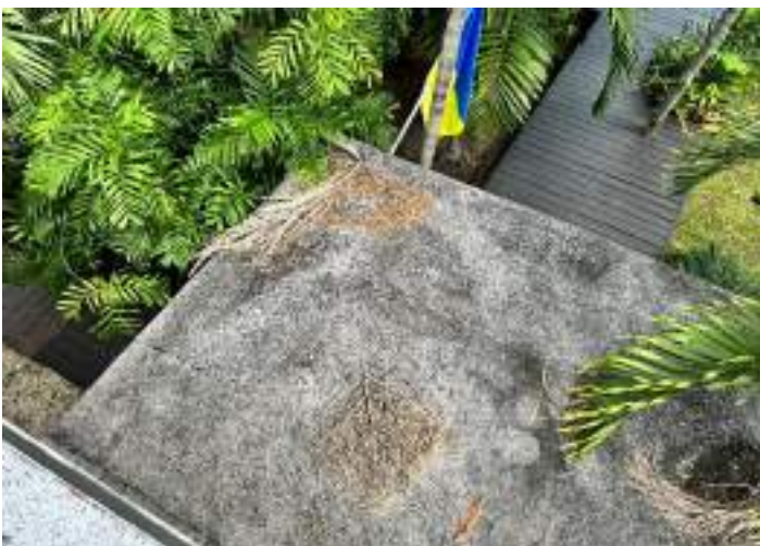
DISCOLORATION/DETERIORATED MEMBRANE
