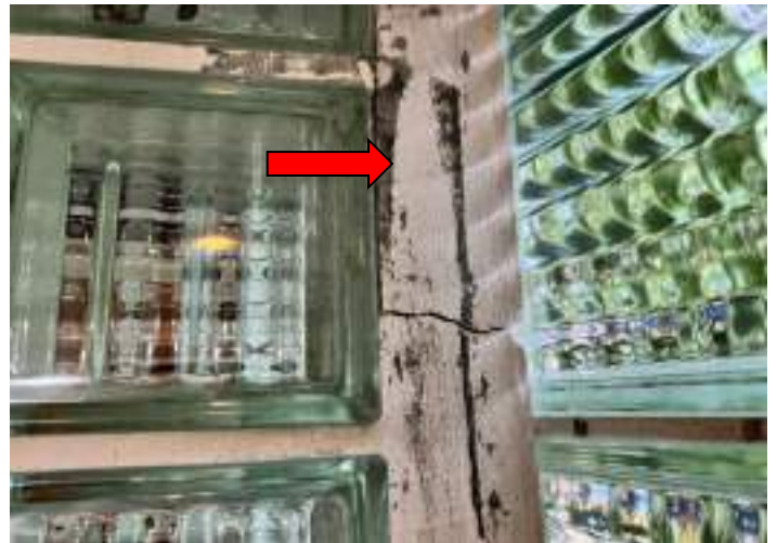
DETERIORATED/MISSING GROUT
