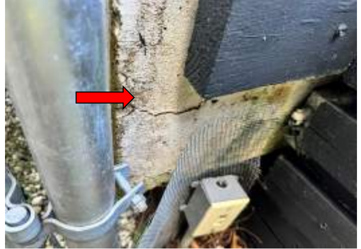
STRUCTURAL SETTLEMENT/CRACKING
