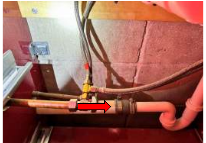
PLUMBING DETAIL/RUBBER HUB CONNECTOR
