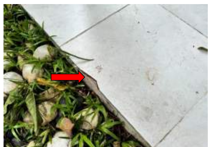
CRACKED/DAMAGED TILE
