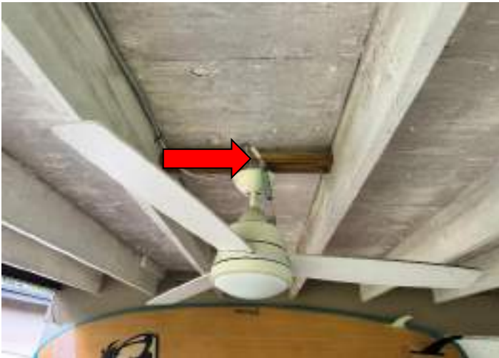
EXPOSED WIRES
