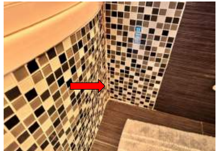
MISSING/DETERIORATED CAULK
