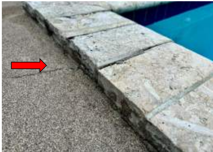
SETTLEMENT CRACKS
