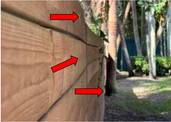
WARPED FENCE
