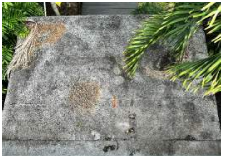
DISCOLORATION/DETERIORATED MEMBRANE
