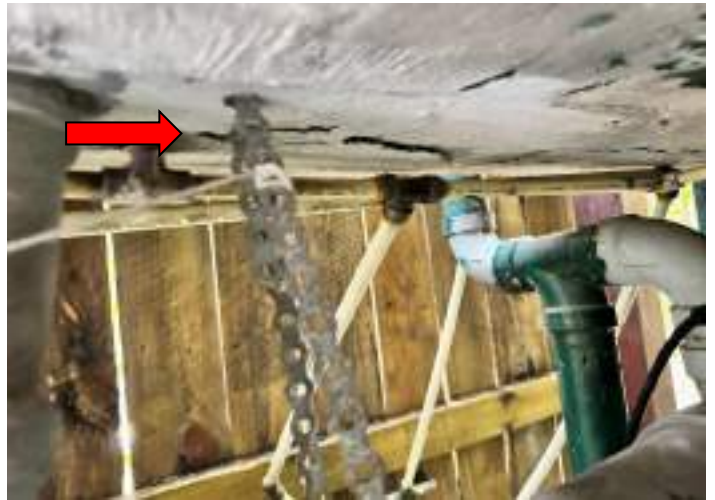
SPALLING/EXPOSED REBAR
