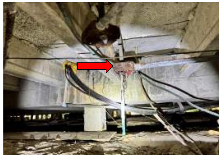
EXPOSED WIRES
