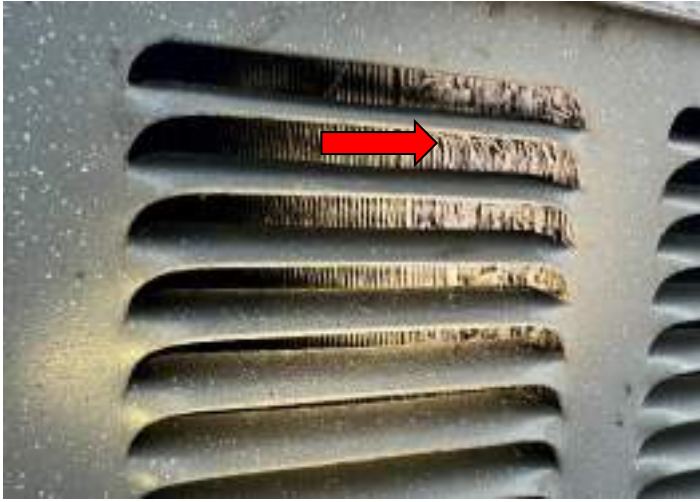
DAMAGED COIL
