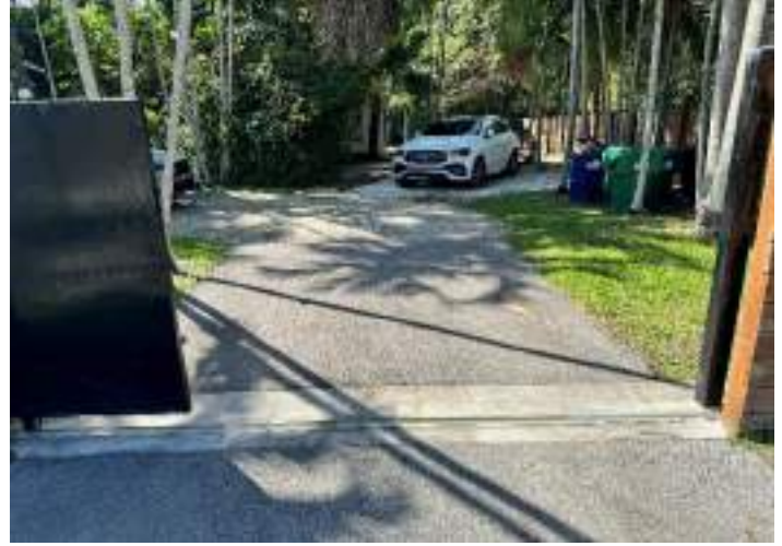
MAIN GATE OPERATIONAL
