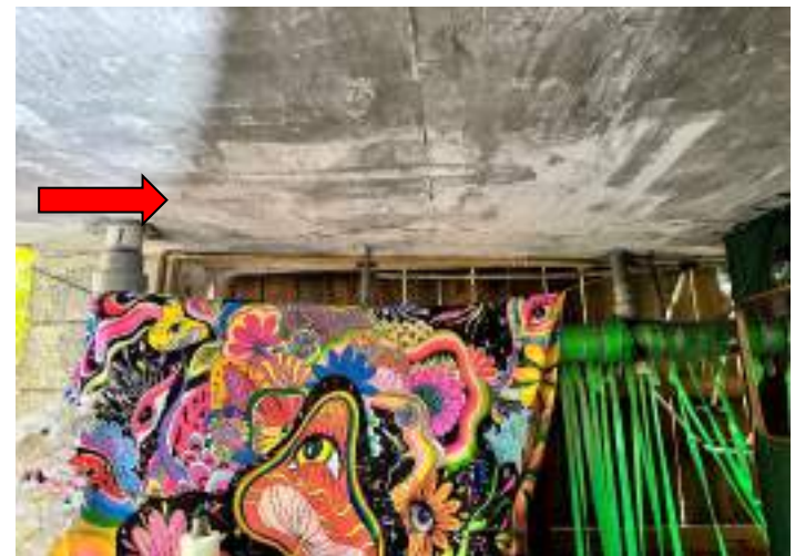
SPALLING/EXPOSED REBAR
