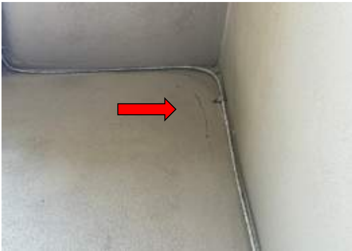
HAIRLINE CRACKS
