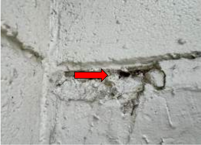
EXPOSED REBAR
