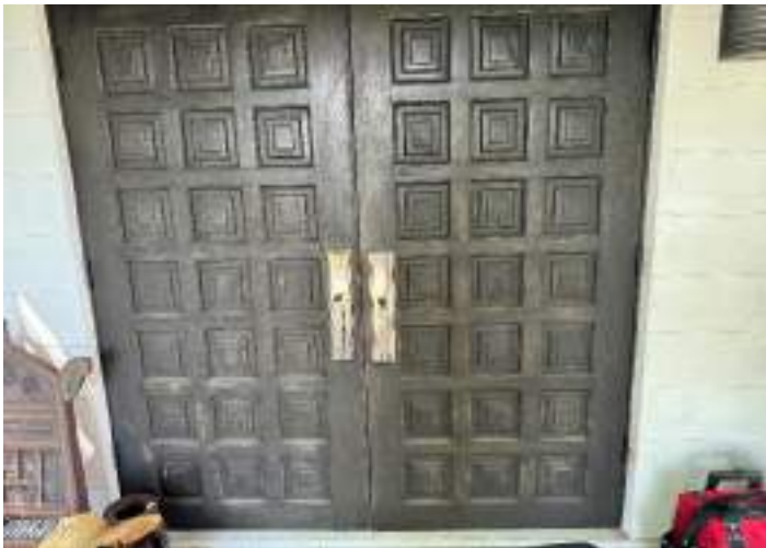
MAIN ENTRY DOOR
