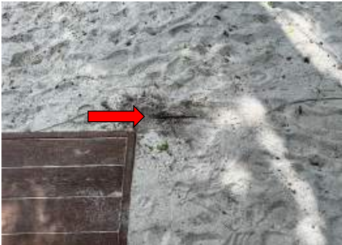
EXPOSED WIRES
