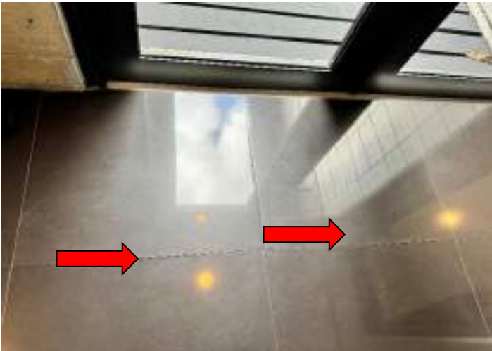
DETERIORATED/MISSING GROUT
