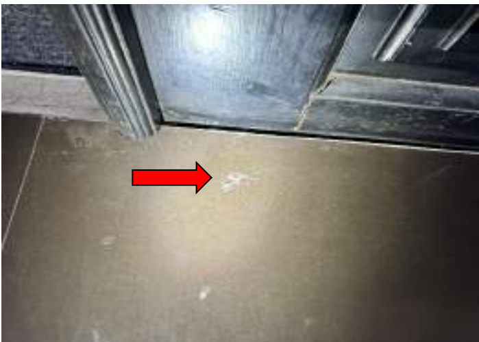
CRACKED/DAMAGED TILE
