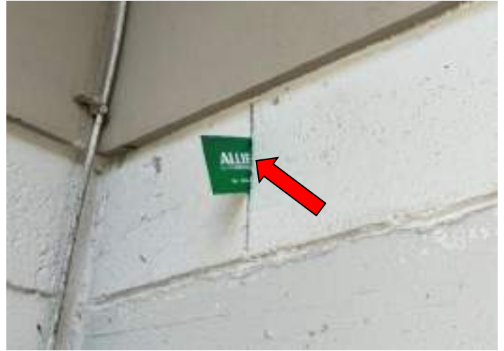
MISSING GROUT/CEMENT
