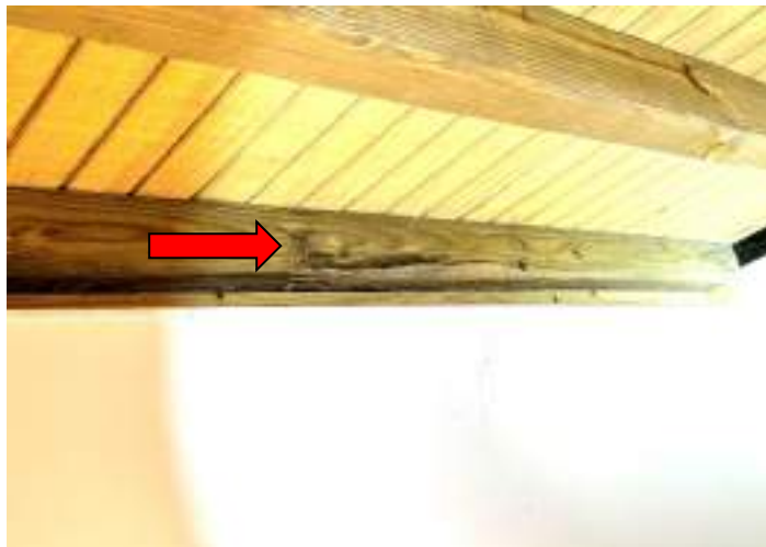
DAMAGED RAFTER
