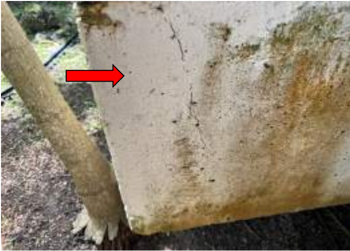
STRUCTURAL SETTLEMENT/CRACKING
