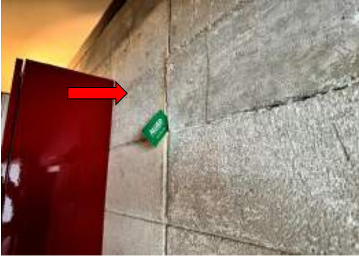
DETERIORATED/MISSING GROUT
