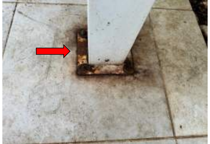
RUST/CORROSION
