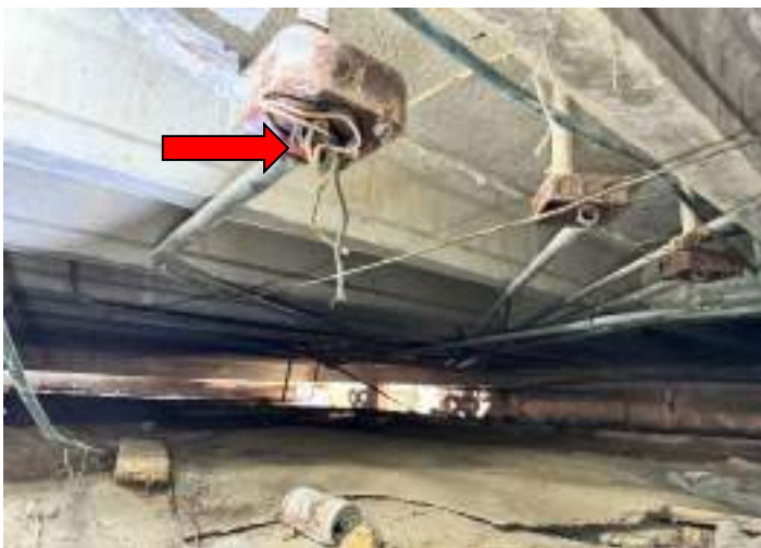
EXPOSED WIRES
