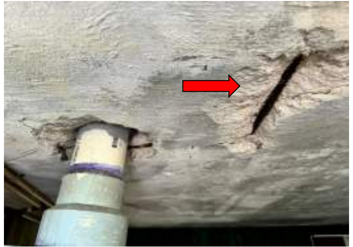
SPALLING/EXPOSED REBAR
