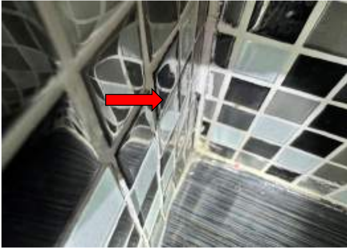
MISSING/DETERIORATED CAULK
