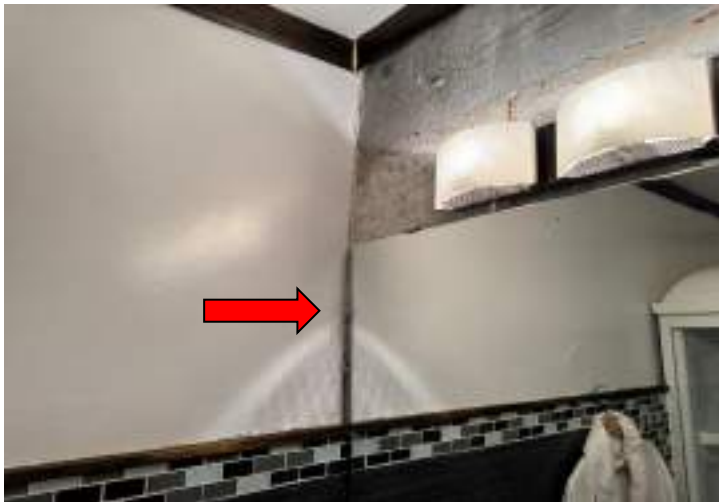
EXPOSED WIRES
