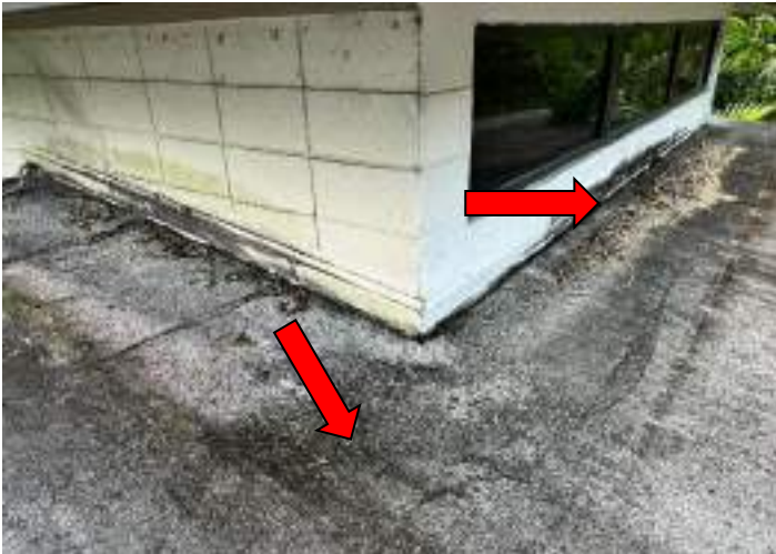
DISCOLORATION/DETERIORATED MEMBRANE
