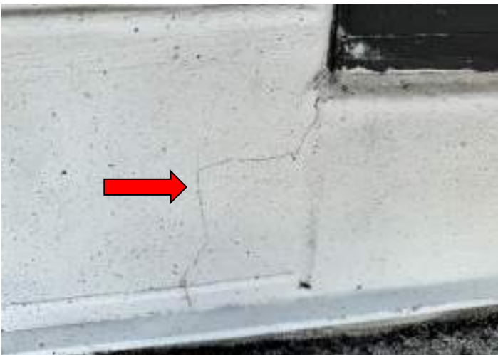
HAIRLINE CRACKS
