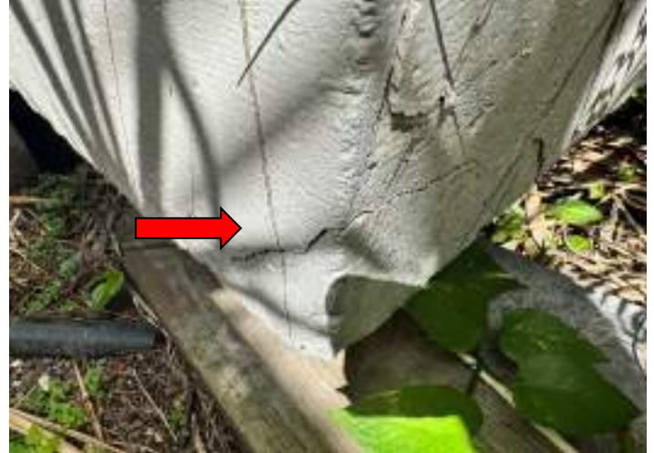
STRUCTURAL SETTLEMENT/CRACKING
