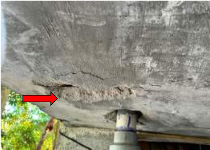
SPALLING/EXPOSED REBAR
