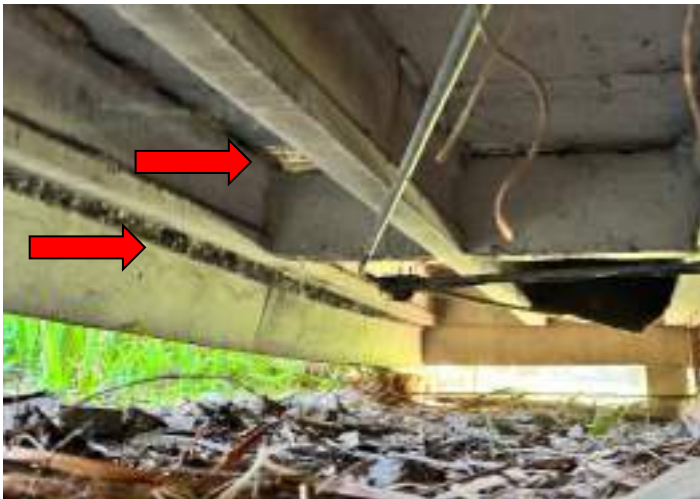
SPALLING/EXPOSED REBAR/BULGES/SETTLEMENT
