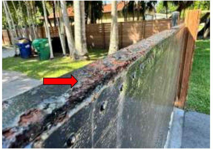
RUST/CORROSION
