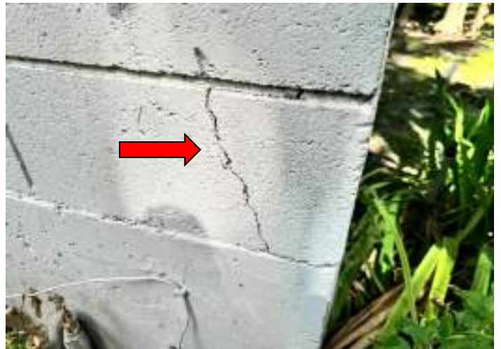
STRUCTURAL SETTLEMENT/CRACKING
