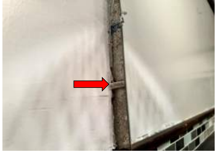
EXPOSED WIRES
