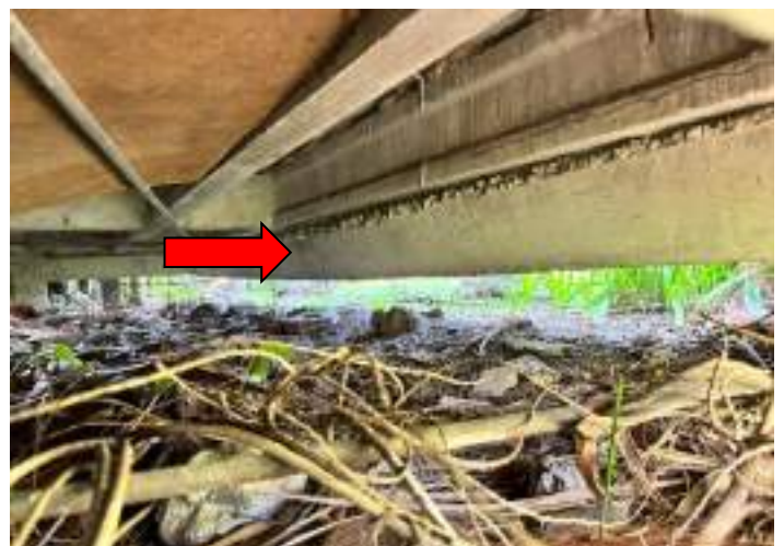
SPALLING/EXPOSED REBAR/BULGES/SETTLEMENT
