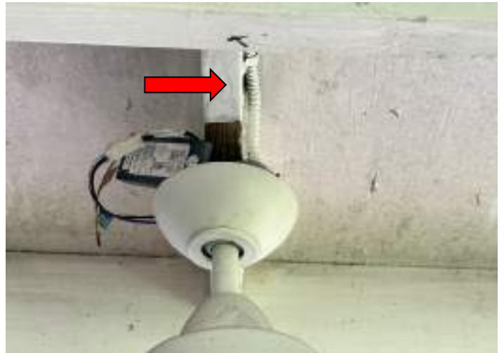
EXPOSED WIRES
