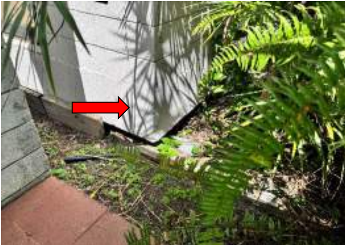
STRUCTURAL SETTLEMENT/CRACKING
