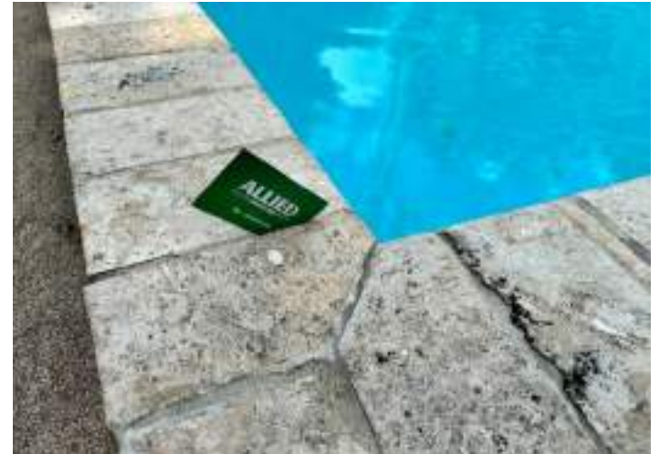
DETERIORATED/MISSING GROUT
