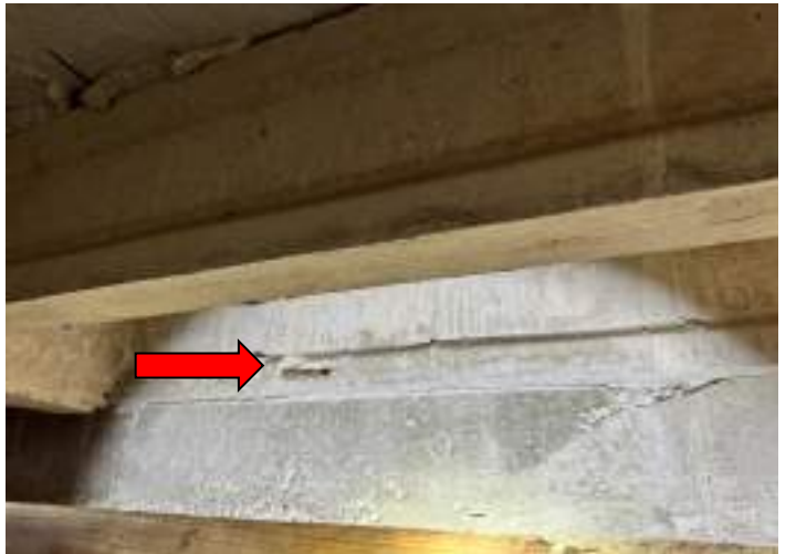
SPALLING/EXPOSED REBAR
