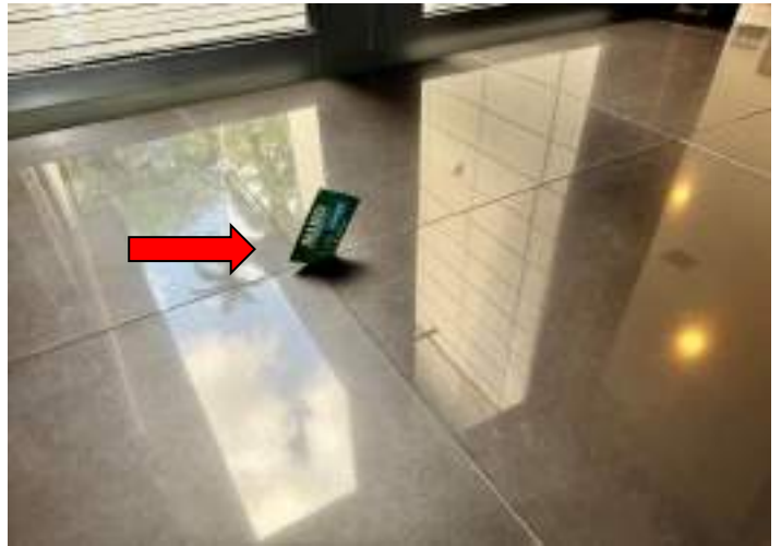
DETERIORATED/MISSING GROUT
