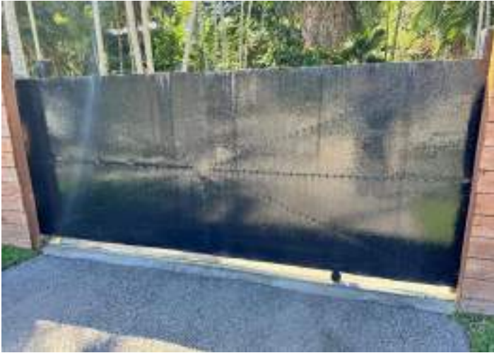
MAIN GATE OPERATIONAL
