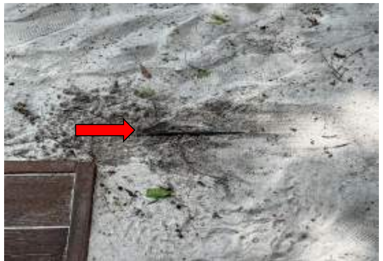
EXPOSED WIRES
