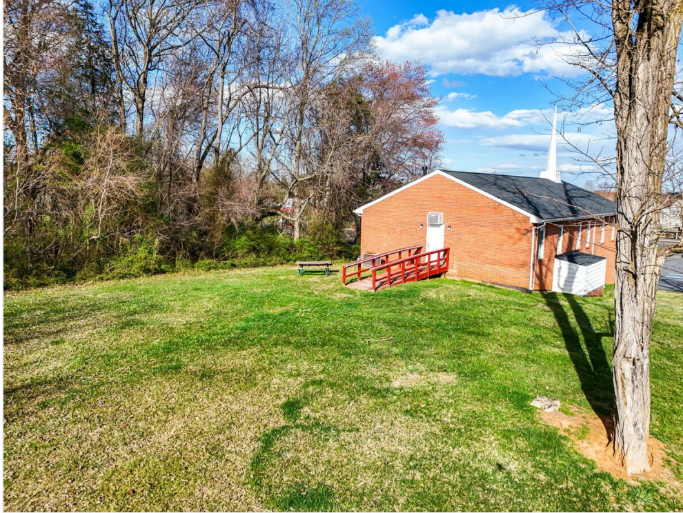
rear entrance / handicap ramp
