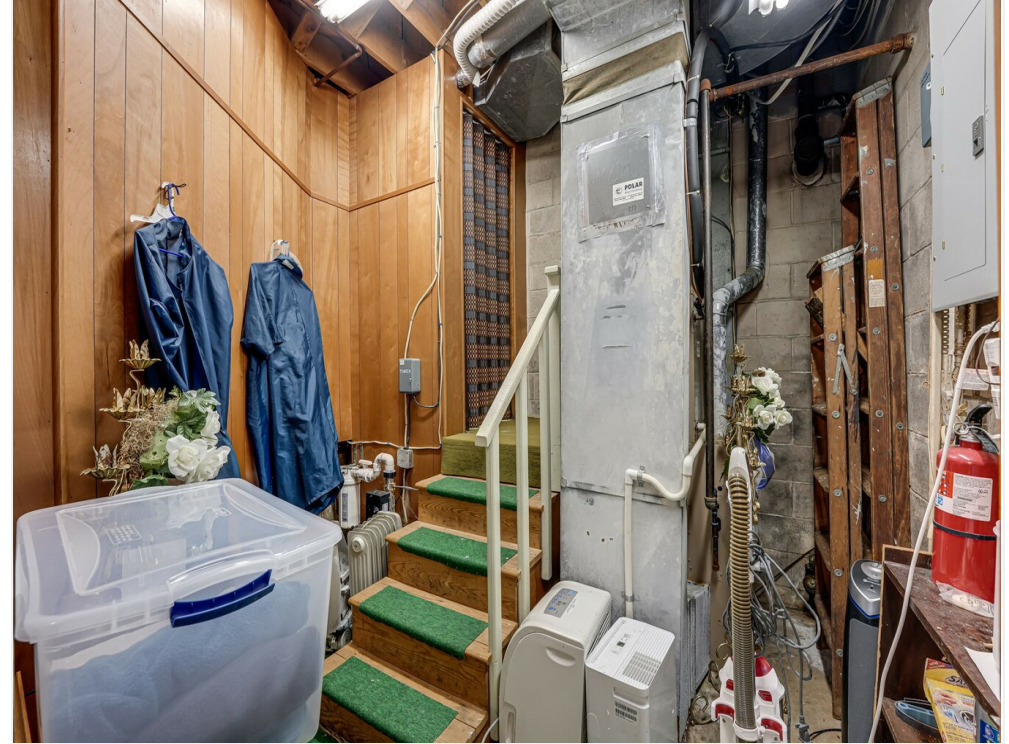
Utility closet /baptismal entrance
