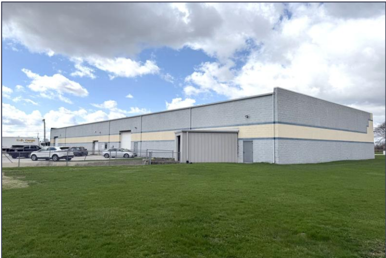
Rear view - Dock
