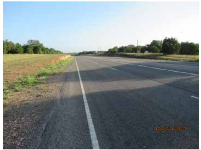
Viewing north along US Highway 281.
