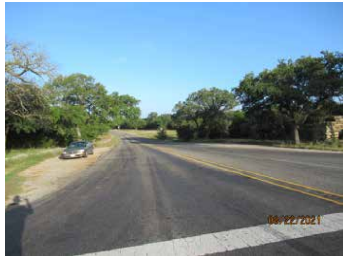
Viewing west along Park Road 4.
