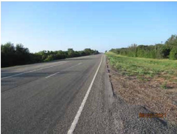
Viewing south along US Highway 281.
