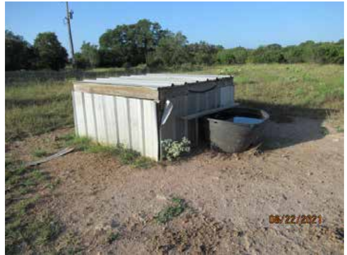
Water well shed located northwest of the house.
