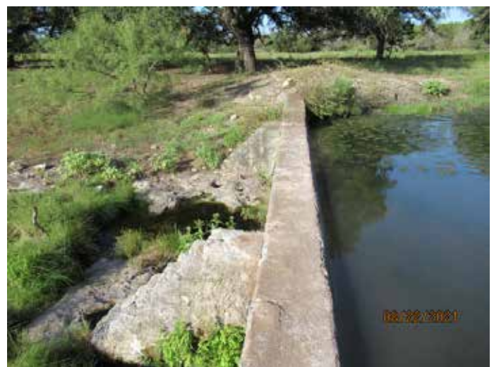
Concrete dam observed on Long Branch 1 Creek.
