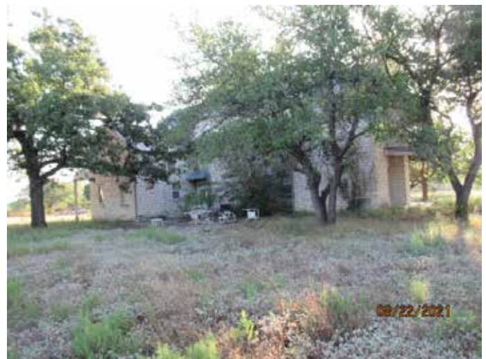
View of west side (rear) of the ranch house.
