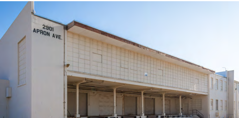
Ground-Level View: Dock-High Doors
