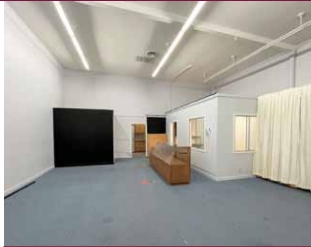
552 S. Murphy Avenue - Interior
