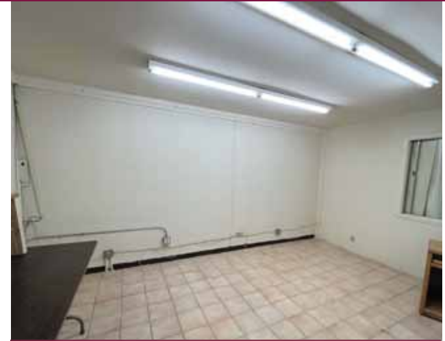
552 S. Murphy Avenue - Interior
