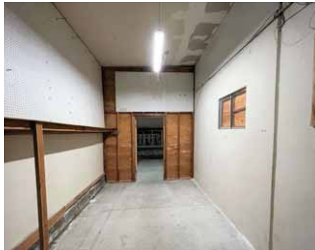
552 S. Murphy Avenue - Interior
