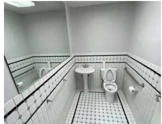
552 S. Murphy Avenue - Interior
