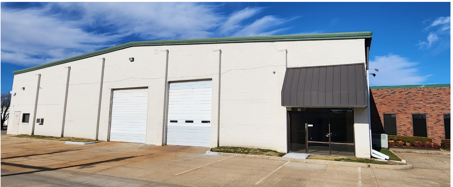
Suite M - Loading/OH Doors
