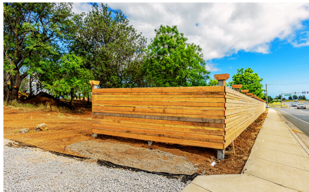
Wood Privacy Entry & Barrier.
