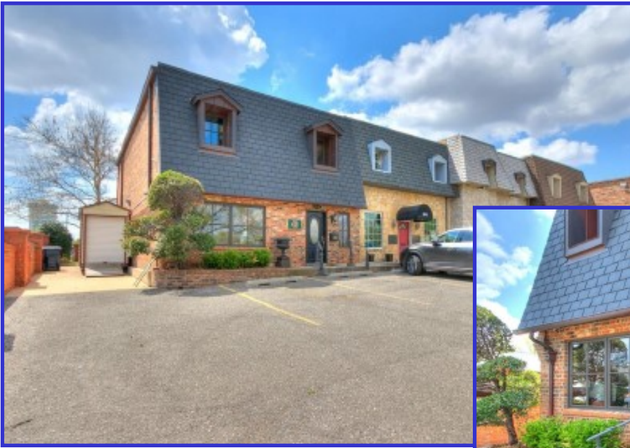
North Side of Building with Main Entry & Parking Lot (Side Storage Unit Included)
