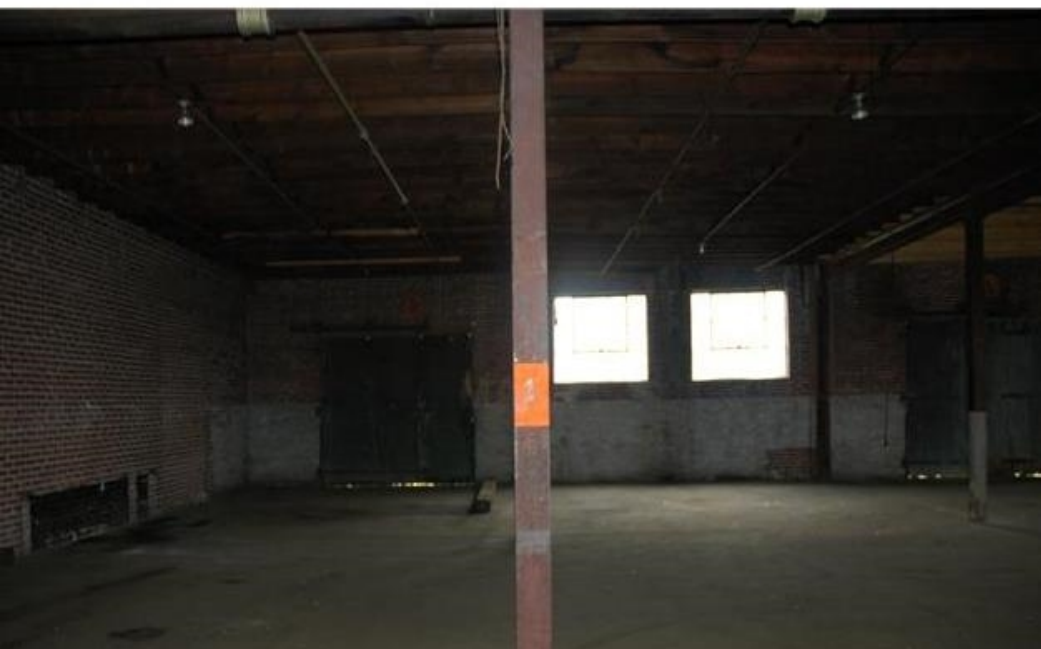
Empty Warehouse Yard Space
