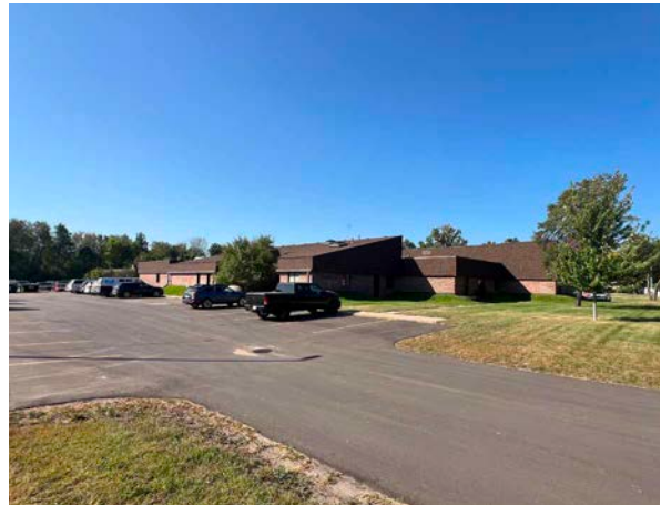
Back/East Side of Building
