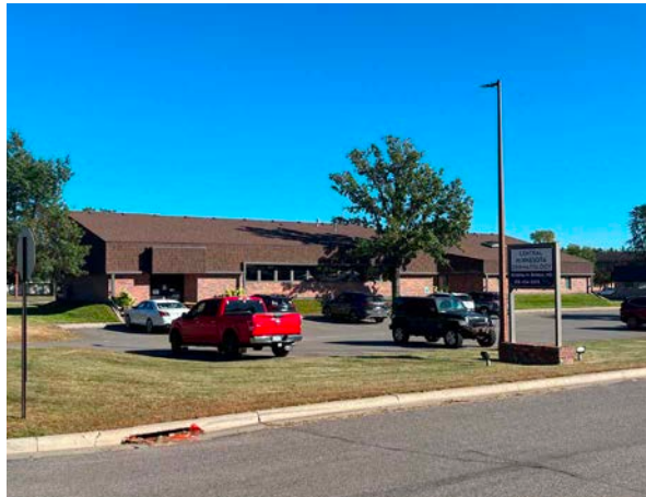
Front/West Side of Building
