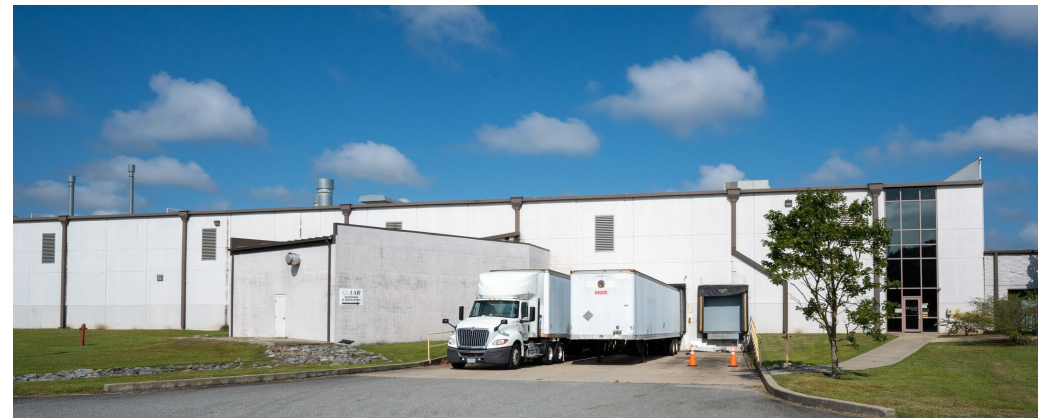
3 LOADING DOCKS AT FRONT OF BUILDING
