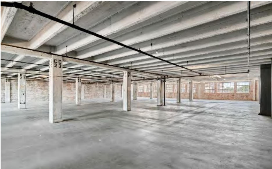
The two adjacent brick buildings are former warehouse storage buildings. The taller building includes concrete flooring, columns, and brick walls (left photos), while the shorter, older building is a wood timber structure with brick walls.
