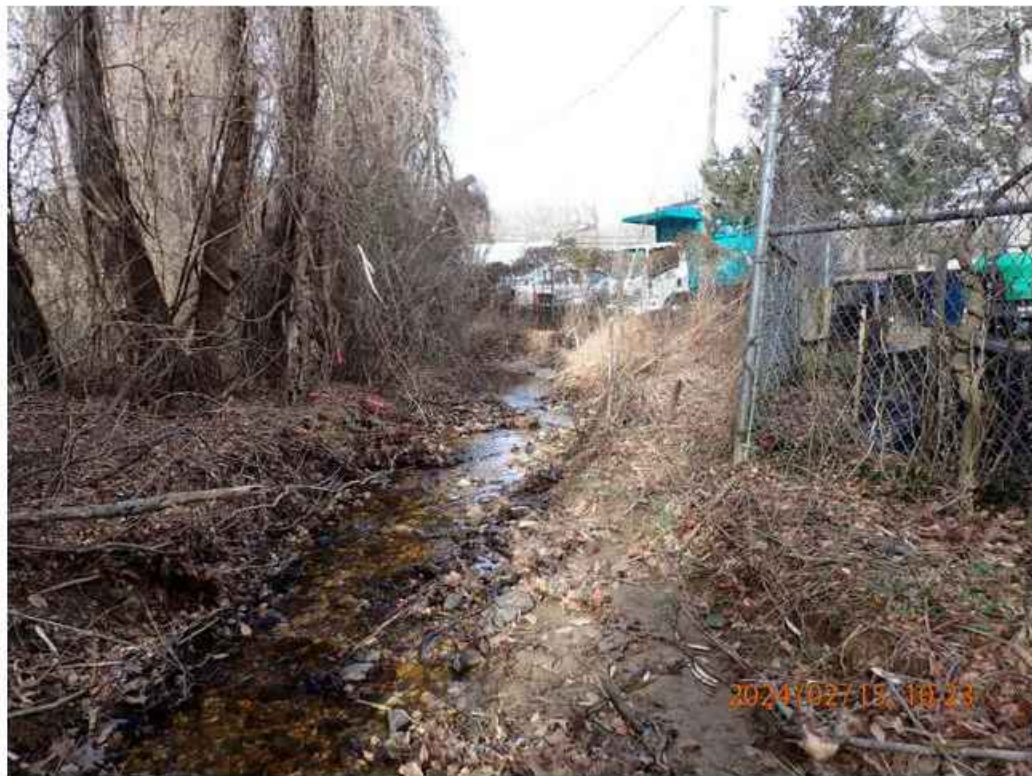
Photo 3 – Facing W, downstream in R3 channel near flag A6.
