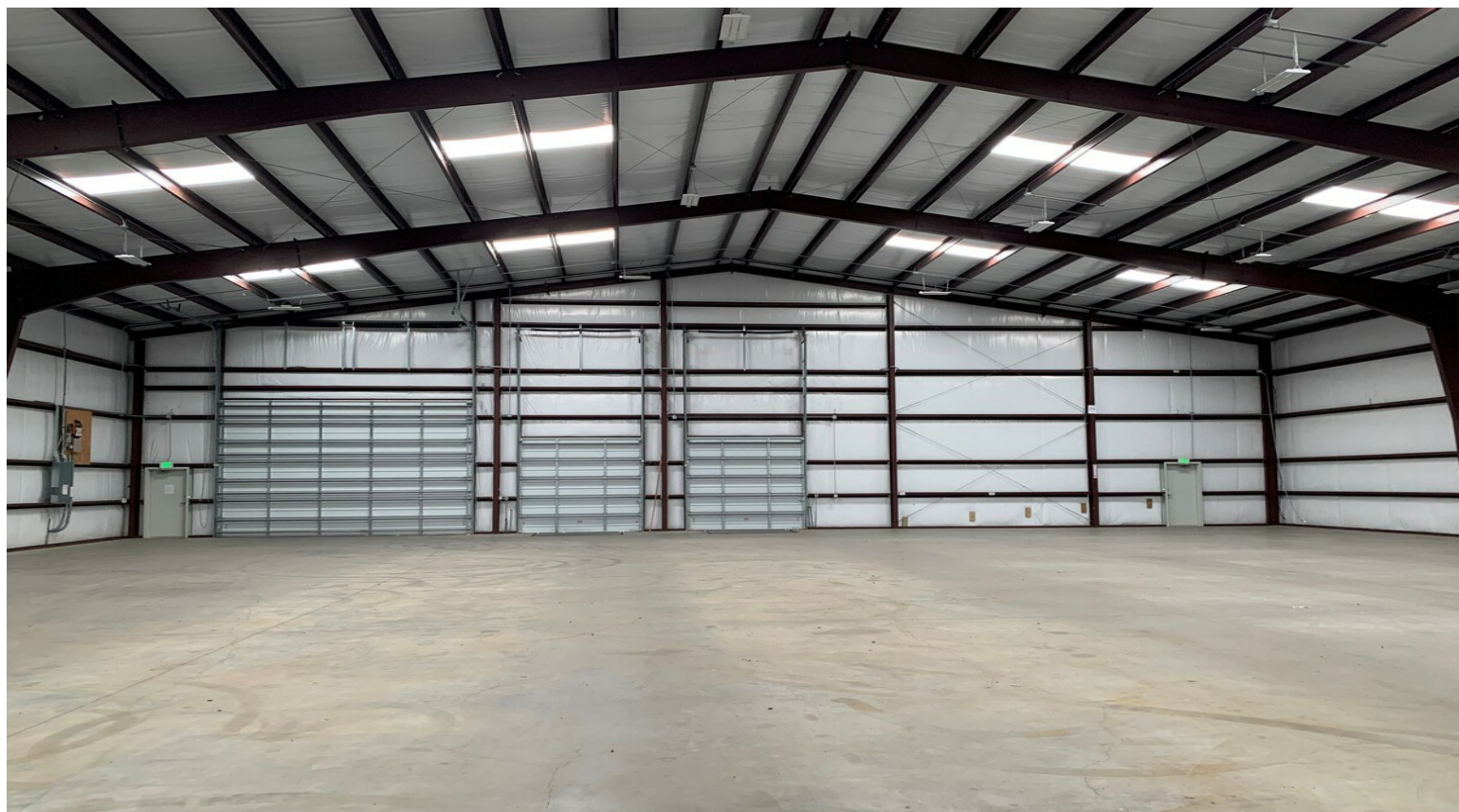
Bldg 2 - T.I. for build out available
