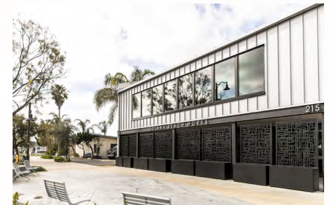
EXTERIOR PATIO FOR SUITE 100
