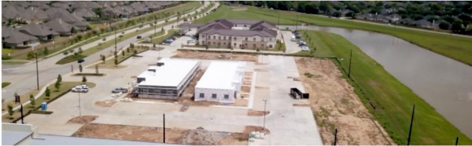
Phase 1 Building A & B - Grand Parkway in the near horizon.
