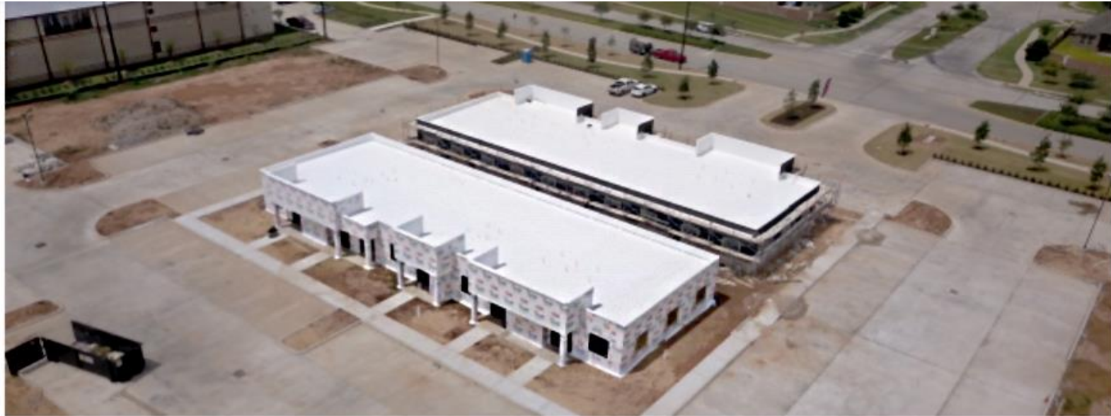
Phase 1 Building A & B - Grand Parkway in the near horizon.
