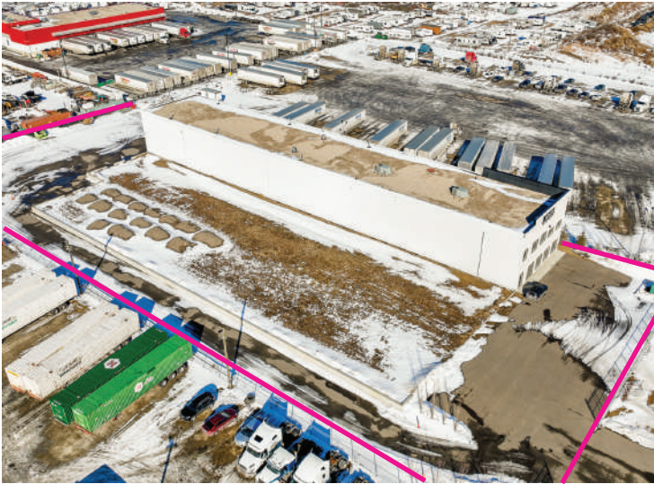
Overview of property
