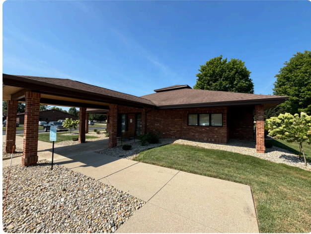
Exterior side view with covered walkway
