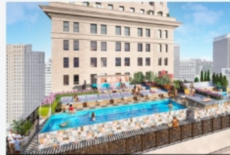
Sky Central Apartment Conversion from Office to Residential
