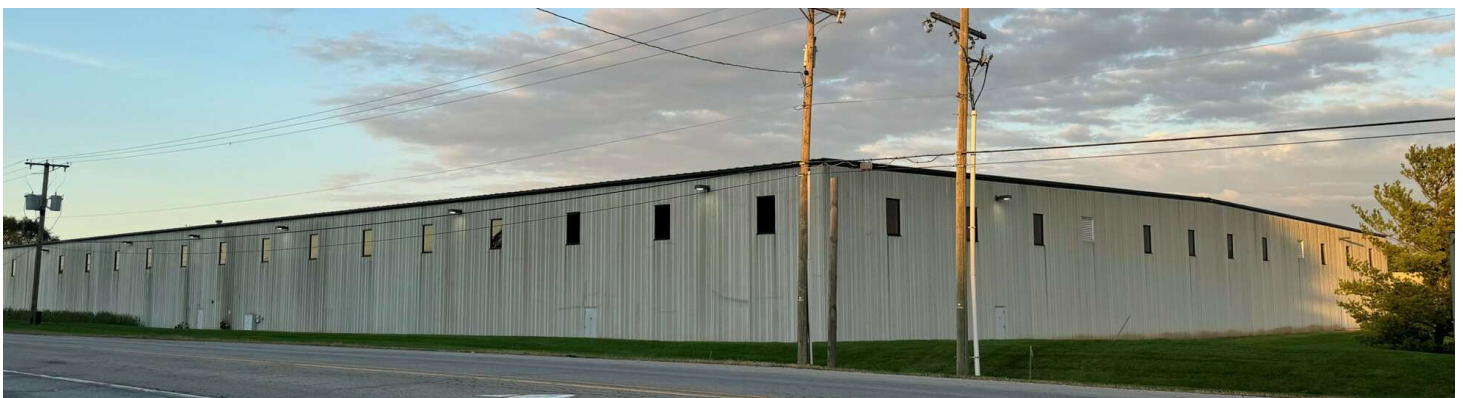
West Side of Building
