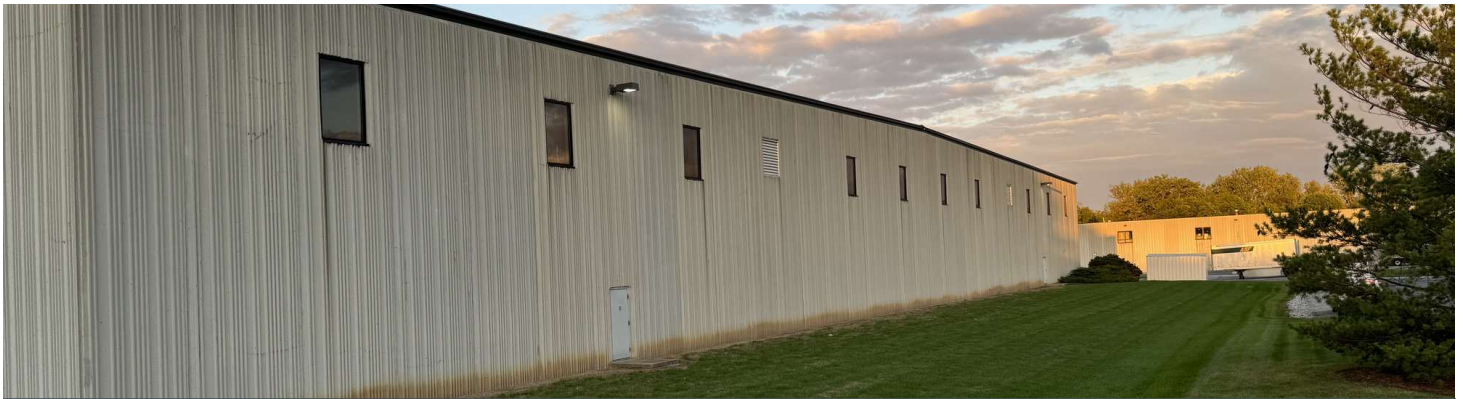
South Side of Building
