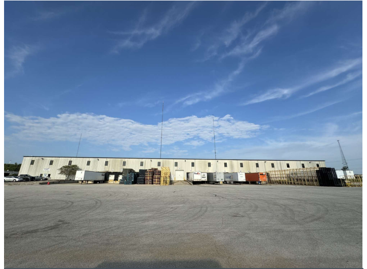
East Side of Building
