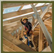
Building Material Supply
