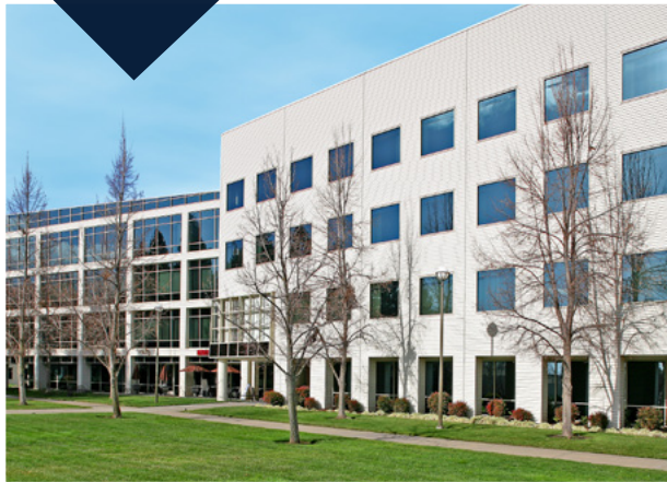
BUILDING A (ASPIRE) 10860 GOLD CENTER DRIVE
