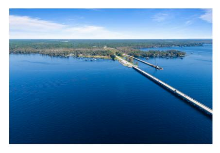
New First Coast Expressway bridge under construction over the St. Johns River just south of where the Shands Bridge stands currently. The vertical height clearance of the new bridge will be 65 feet. The additional 20 feet of clearance will match the Buckman Bridge's clearance to the north removing all barriers for marine traffic.
