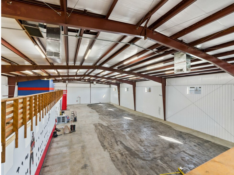
110 Yale Ln Bldg A
